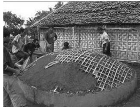
Figure 11. Stages of Cubang Construction for Typical Hamlet Family of 5 People
